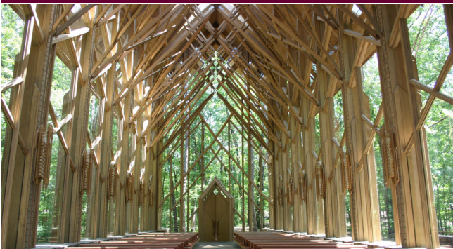
An interior view of the Anthony Chapel.
